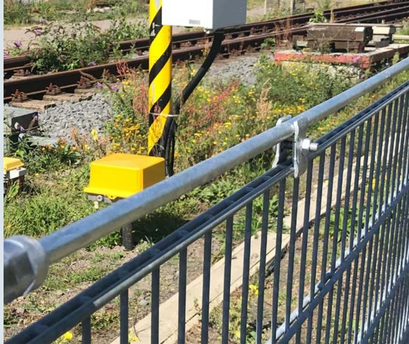
Short-circuit wire on a noise barrier or grating fence
