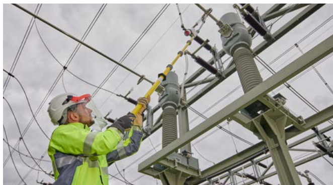
PHE4 voltage detector applied in a 110 kV outdoor switching station.
