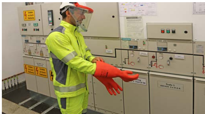
Work on live parts with insulating gloves.
