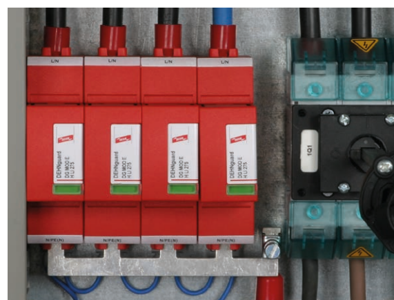
Figure 9 DEHNGuard SE H LI = surge arrester with integrated "Lifetime Indication" early warning system
