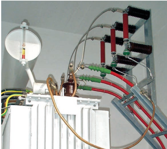
Figure 10 DEHNmid: surge arrester for medium-voltage systems
